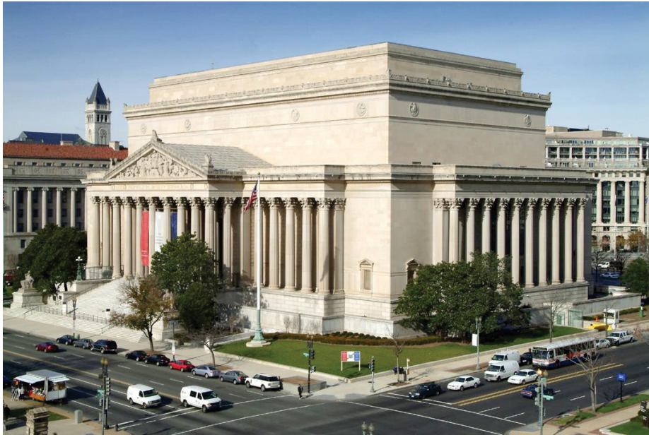
National Archives Building Washington, DC
