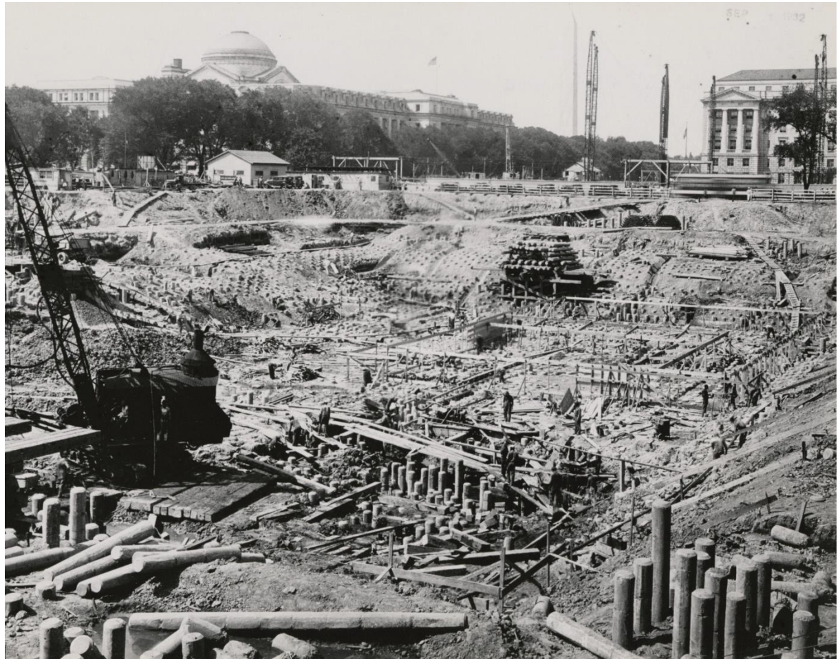
Construction of the Foundation for the National Archives Building, September 1, 1932
